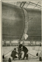
Near View of the Space Between the Two Halves of the Envelope, Showing the Propeller Which Drives It.
